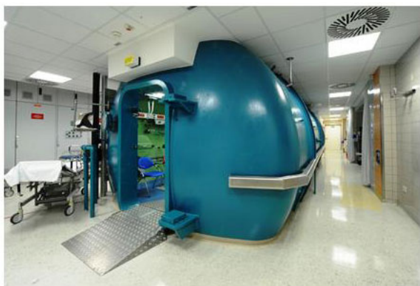
Figure 4. Multiplace-Hyperbaric chamber for emergency HBO.
